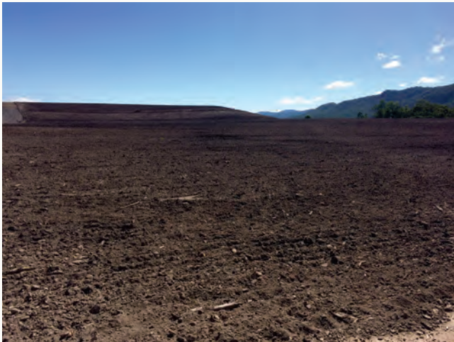
Plate 3: Growth Medium Development – Topsoil Spreading
