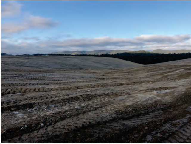
Plate 1: Landform Establishment – Bulk Shaping
