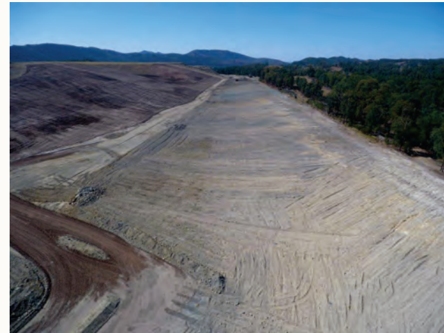
Plate 2: Landform Establishment – Bulk Shaping and Topsoil Spreading
