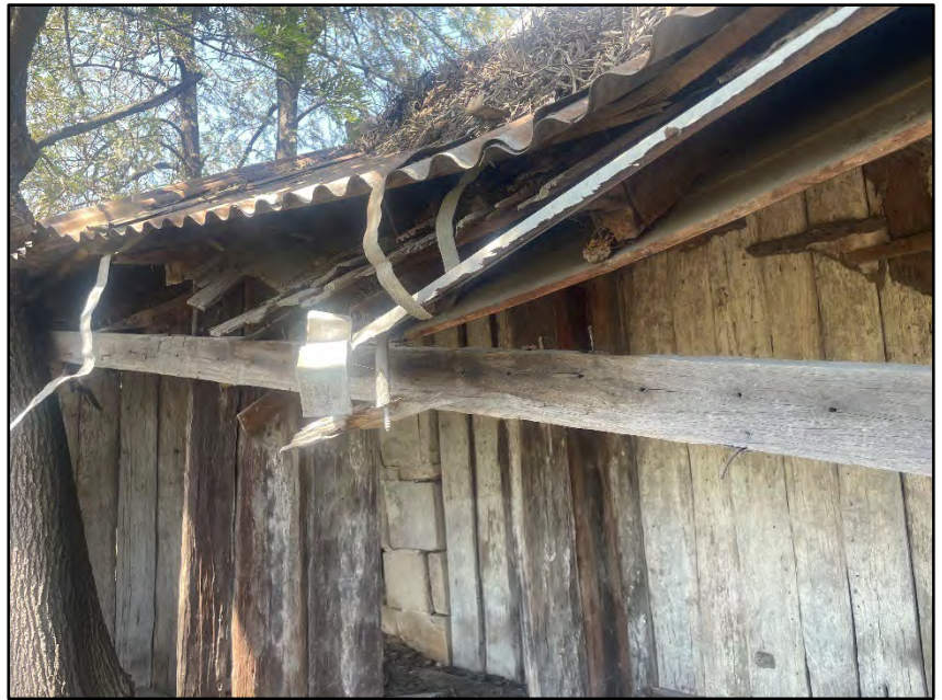
Increased slumping along eastern wall
