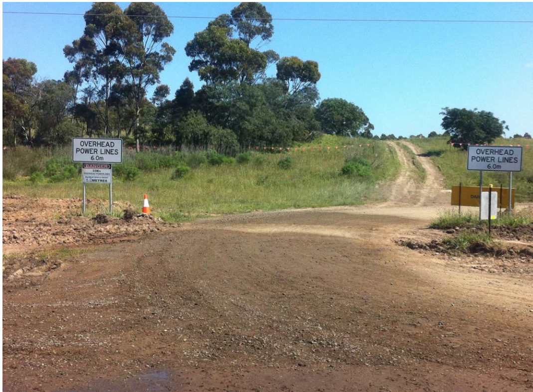
Figure 6: 33kV power line clearance signs located at the entrance of Macquarie Generation access road (turn from the Brunkers Lane) prior to LW7B start.
