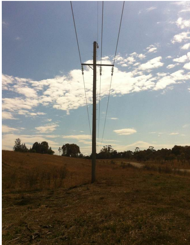
Figure 4: 33kV power line (PP34) parallel to Maingate 8 in LW7B looking north post-undermining (18/09/12). Rollers were fitted to this line prior to undermining.
