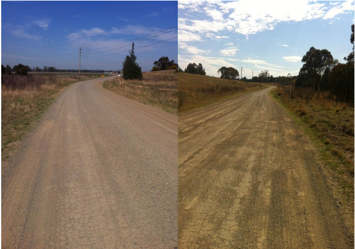
Figure 8: Macquarie Generation access road above LW7B following remediation.
