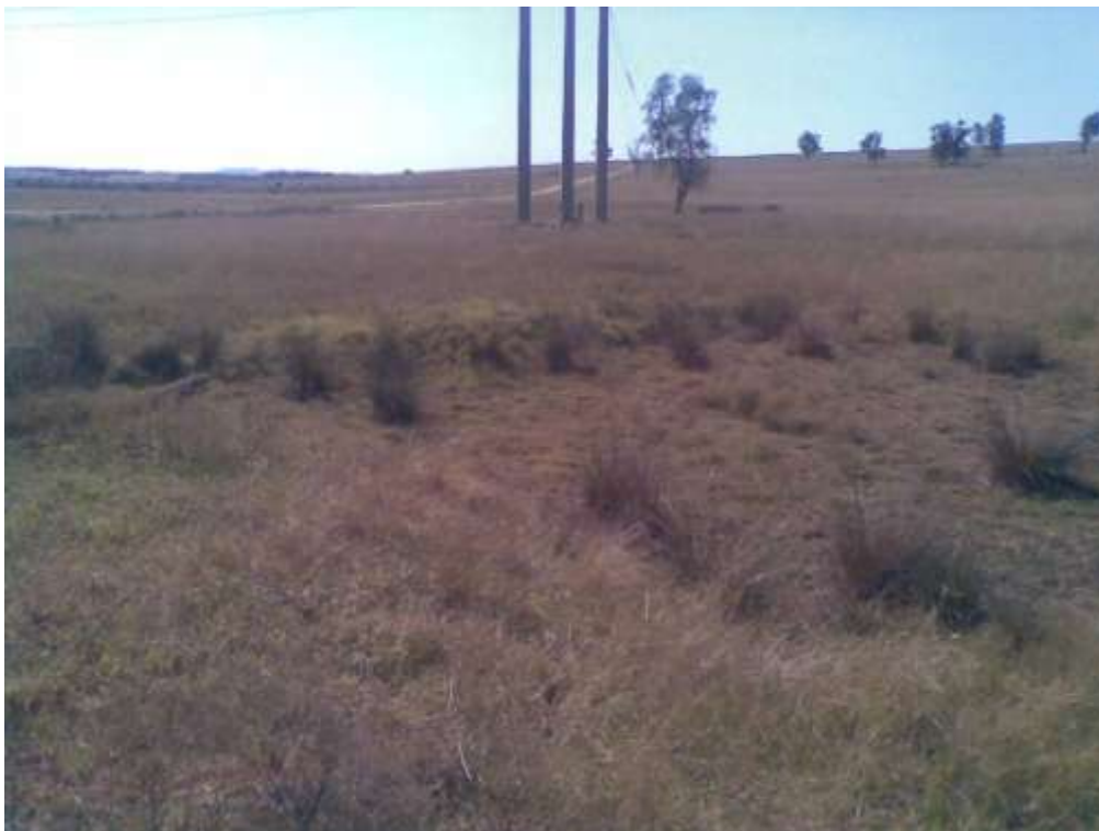
Figure 12: 3 pole power line structure (background) and subsided area (foreground) before significant rain events. Image looking north-west on 30/04/10.
