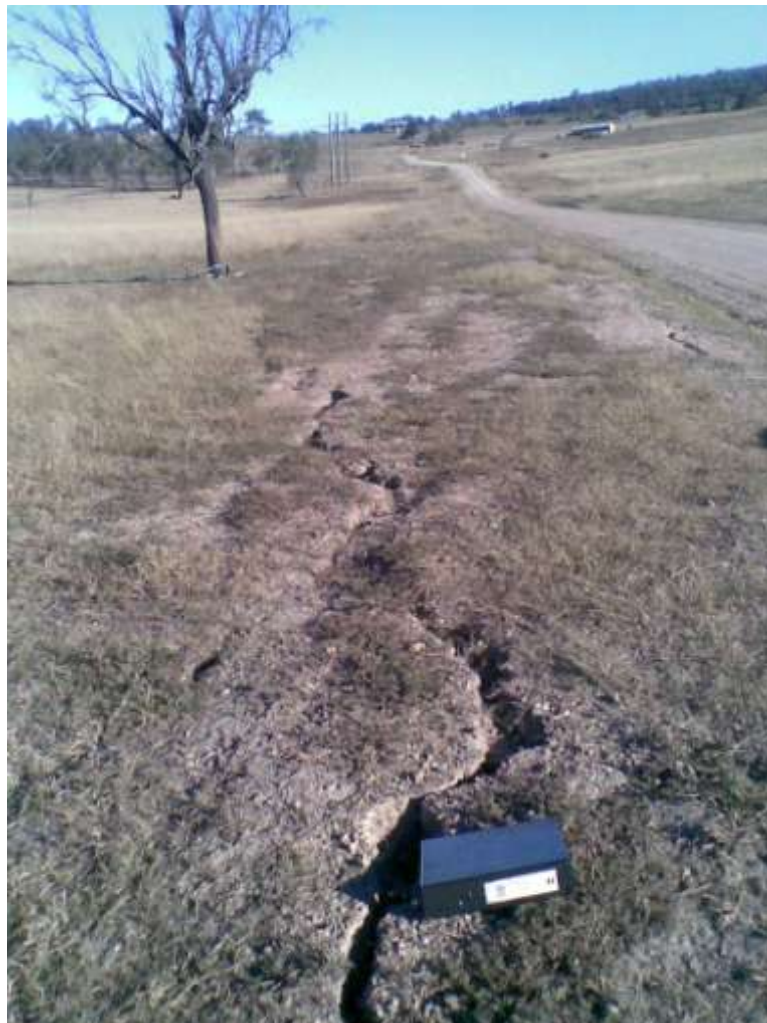
Figure 10: Gateroad crack on surface. In the background the 3 pole power line structure can be seen. This image was taken post stays being fitted to the power line on 12/05/10.
