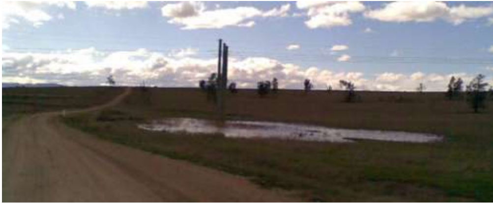
Figure 13: Ponding under Longwall 5 3 pole power line structure on 11/08/10 looking north.
