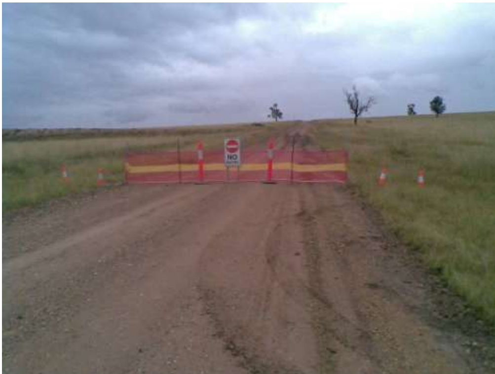
Figure 14: Road barrier which blocked road access whilst road was being undermined.
