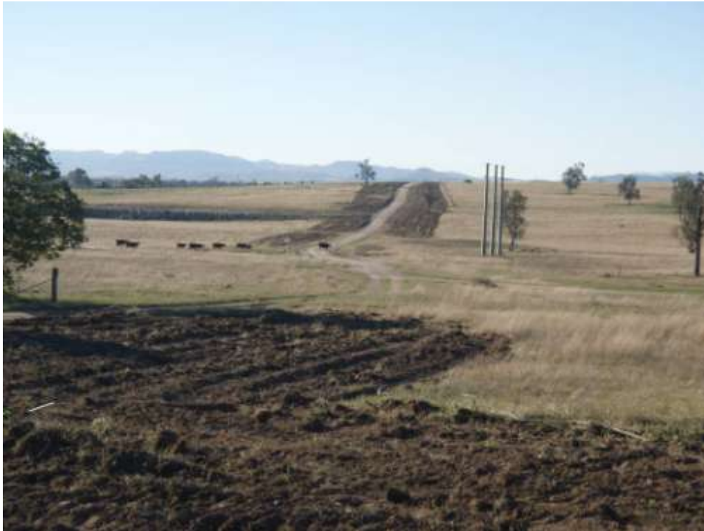
Figure 11: Gateroad cracks post remediation. The ripped section runs the length of visible surface cracks. Image taken looking north. Remediation completed on 25/06/10.
