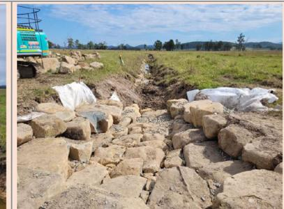
Fig.4 Construction of the rock cascade drop structure
