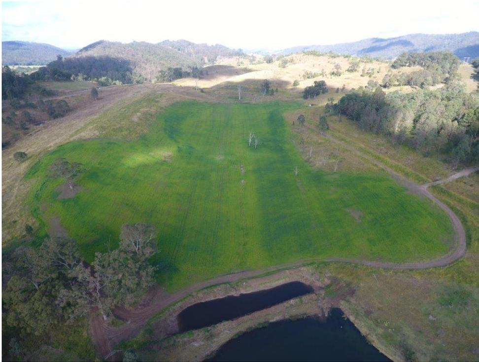
Photo: Shaping and topsoiling completed at Auxiliary Dam 1, Jul
