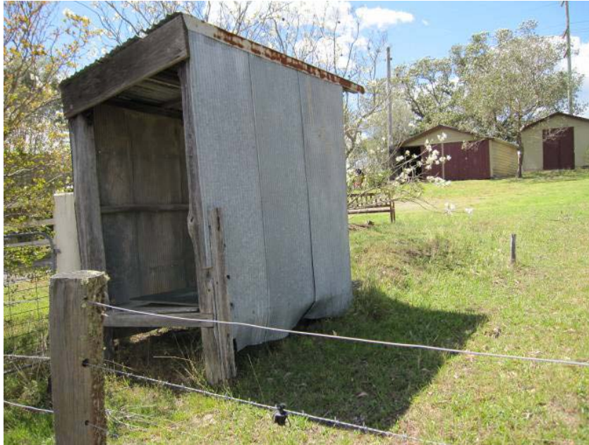
Plate KA-27: Milk shed at front gate
