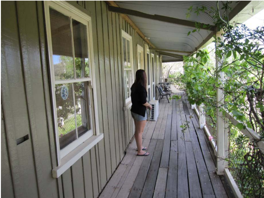
Plate KA-17: Front verandah showing original letter slot on north-west wall
