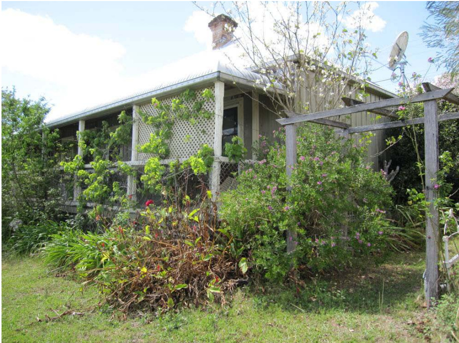
Plate KA-1: Former Weismantels Inn – Facing north-west towards The Bucketts Way
