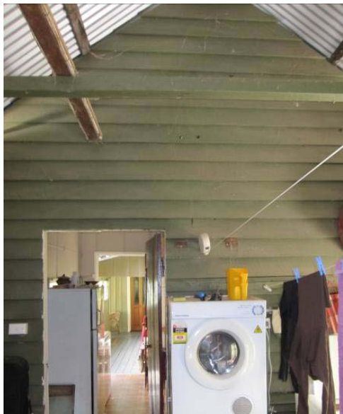
Plate KA-4: Looking north-west from laundry along southern verandah
