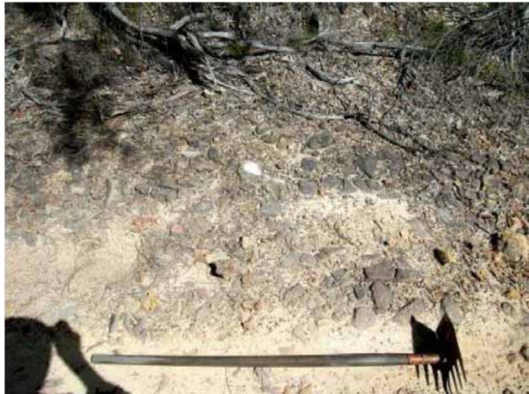
Figure 2.7 Showing coarse aggregate base of the original pavement at Devine's Hill. The surface layer has eroded away (Young 2007: Figure 29)
