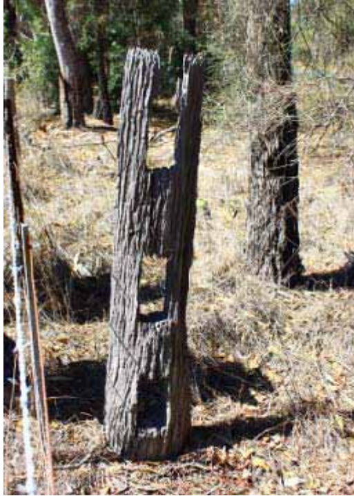
Figure 4.12 Three rail post and rail fence
