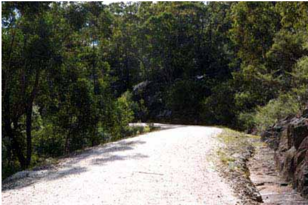
Figure 2.8 Showing pavement and side drains at Devine's Hill section of the Old Great North Road (SEWPaC 2007)
