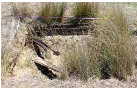
Figure 4.24 Well #2 with timber lining visible
