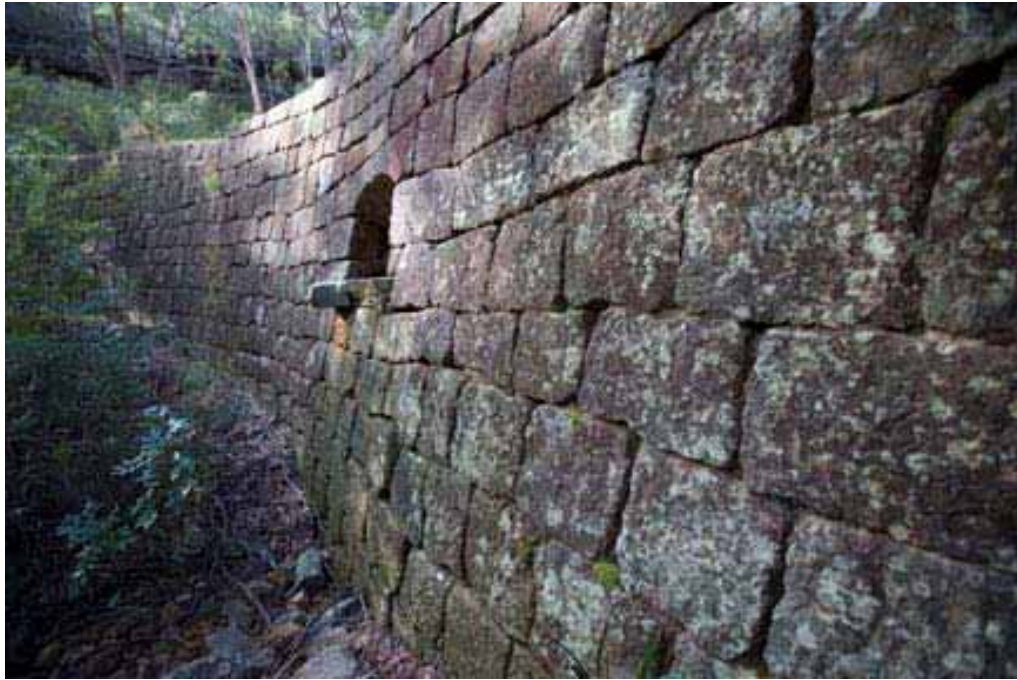
Figure 2.9 Example of retaining wall and culvert, Wiseman's Ferry section of the Old Great North Road (SEWPaC 2007)
