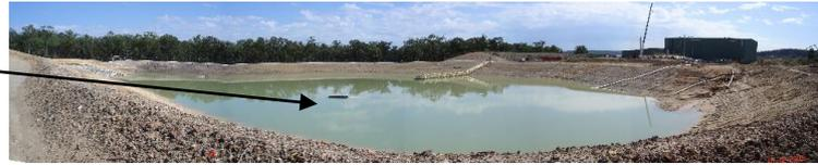
Increased capacity of Moolarben Coal Sediment Dam 106 to collect 100 year ARI flood
