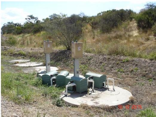
**Plate 5.9.3: Effluent irrigation system adjacent to the application area.**
