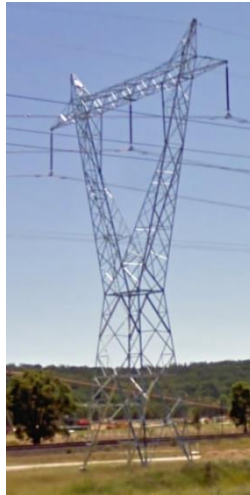
Fig. 6.1 330 kV Suspension Tower
