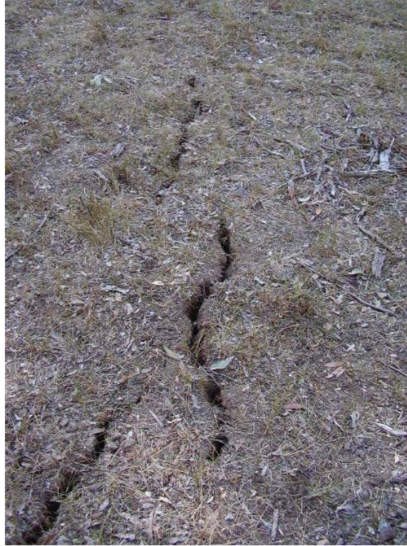
Fig. 4.5 Example of surface tensile cracking in the natural ground surface (observed in the Southern Coalfield at a similar depth of cover as in the Study Area)
