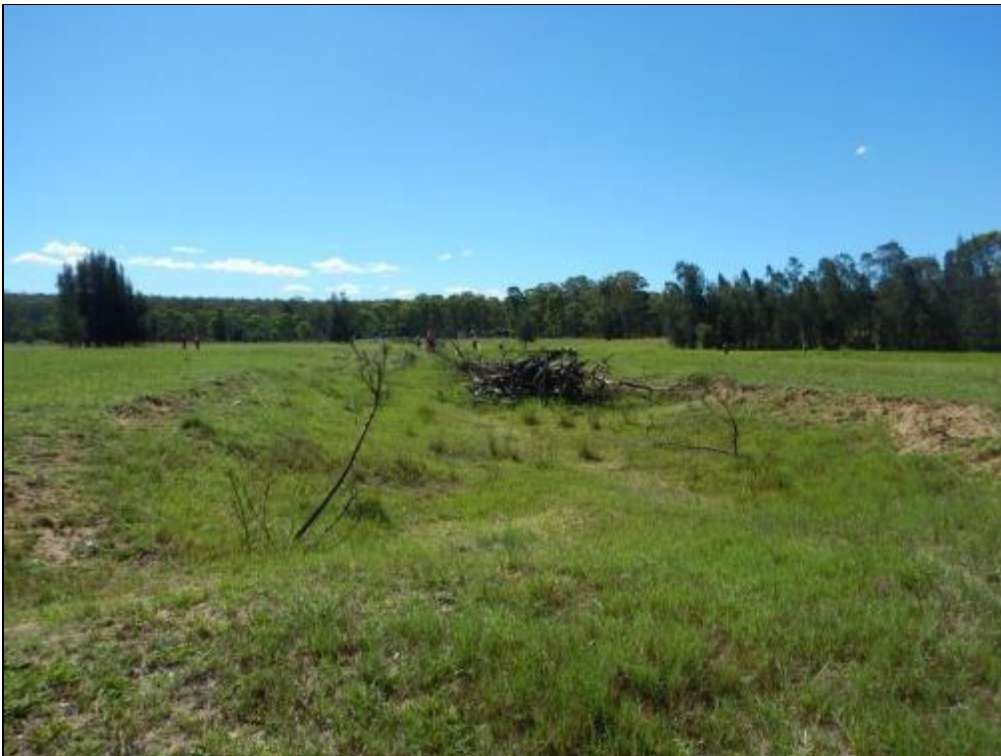
Plate 6 Survey unit 2 showing exposure of alluvium in area of earthworks
