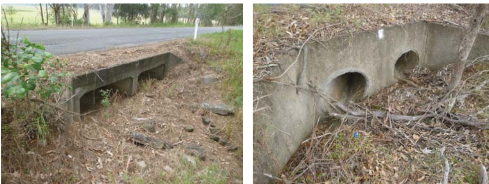
Fig. 6.3 Box culvert SCR-C3 (left side) and concrete culvert SCR-C4 (right side)
