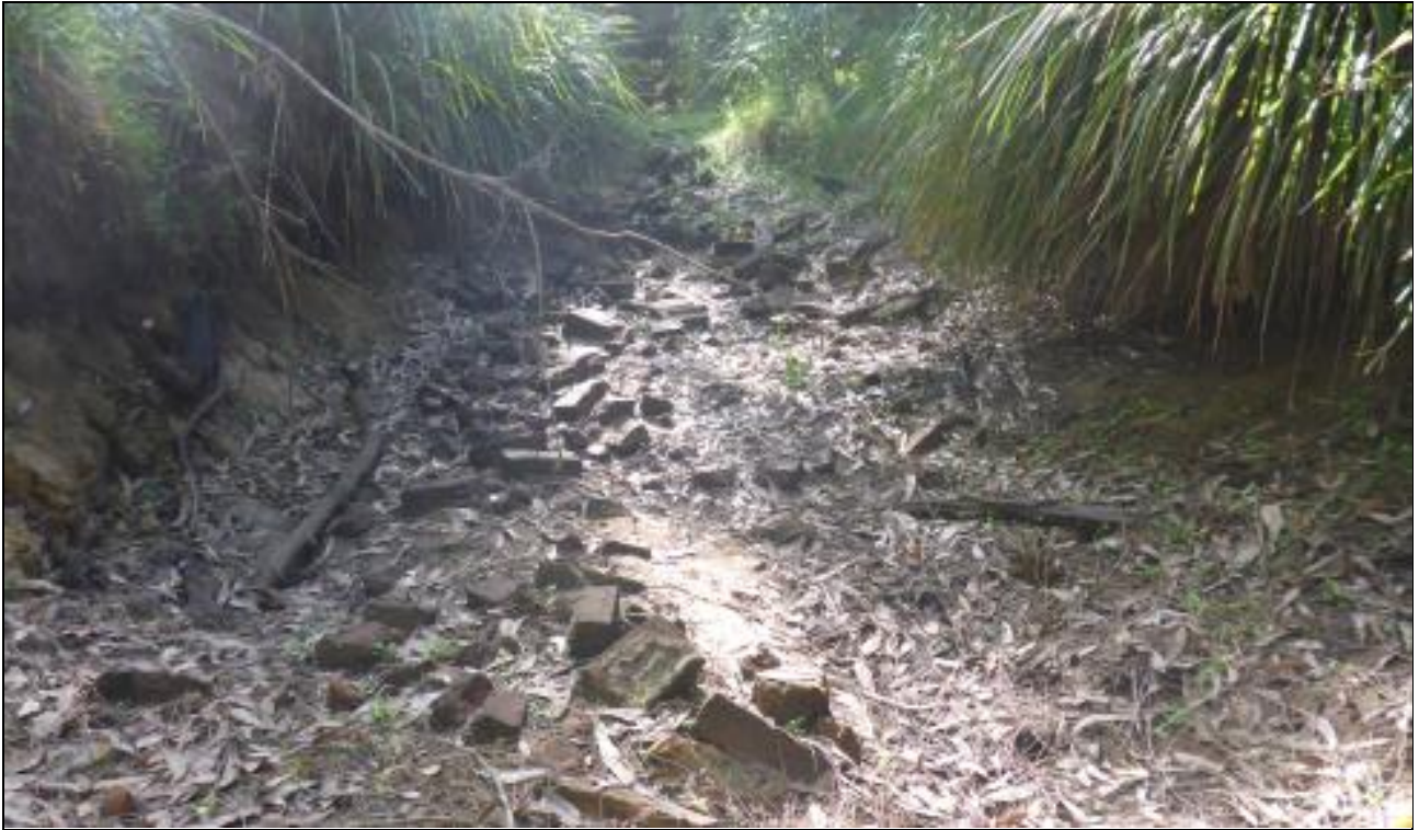
Plate 6.2 View northeast overlooking dam and location of former crossing
