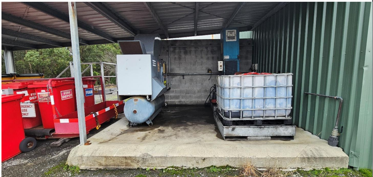
Plate 6: Bunded storage of underground firefighting equipment and IBCs
