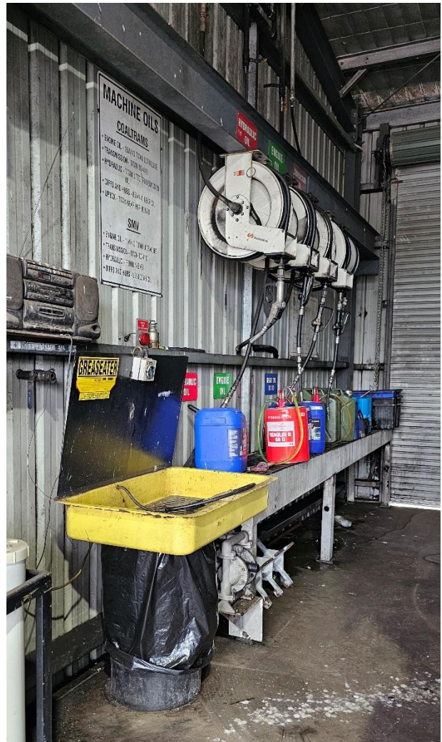
Plate 14: Chemical storage bunding and controlled decanting
