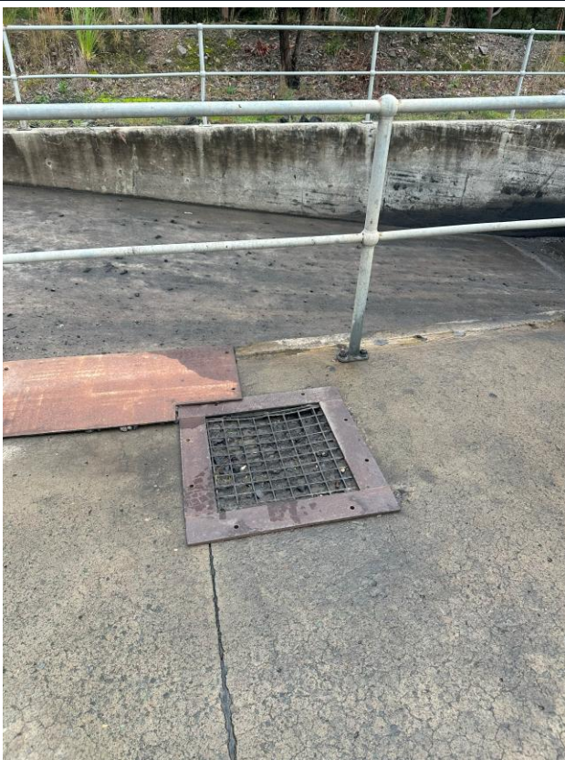
Plate 11: Drain with clogged grate
