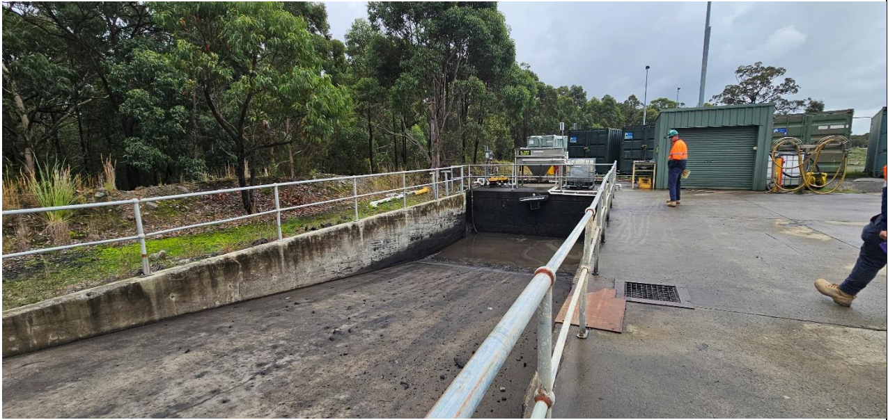
Plate 10: Drain, Sump and Oil/Water Separator
