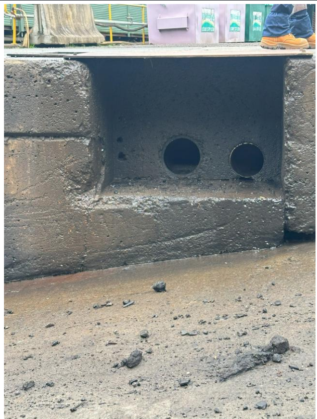
Plate 12: Drainage points from bunding and sump under workshop and hardstand
