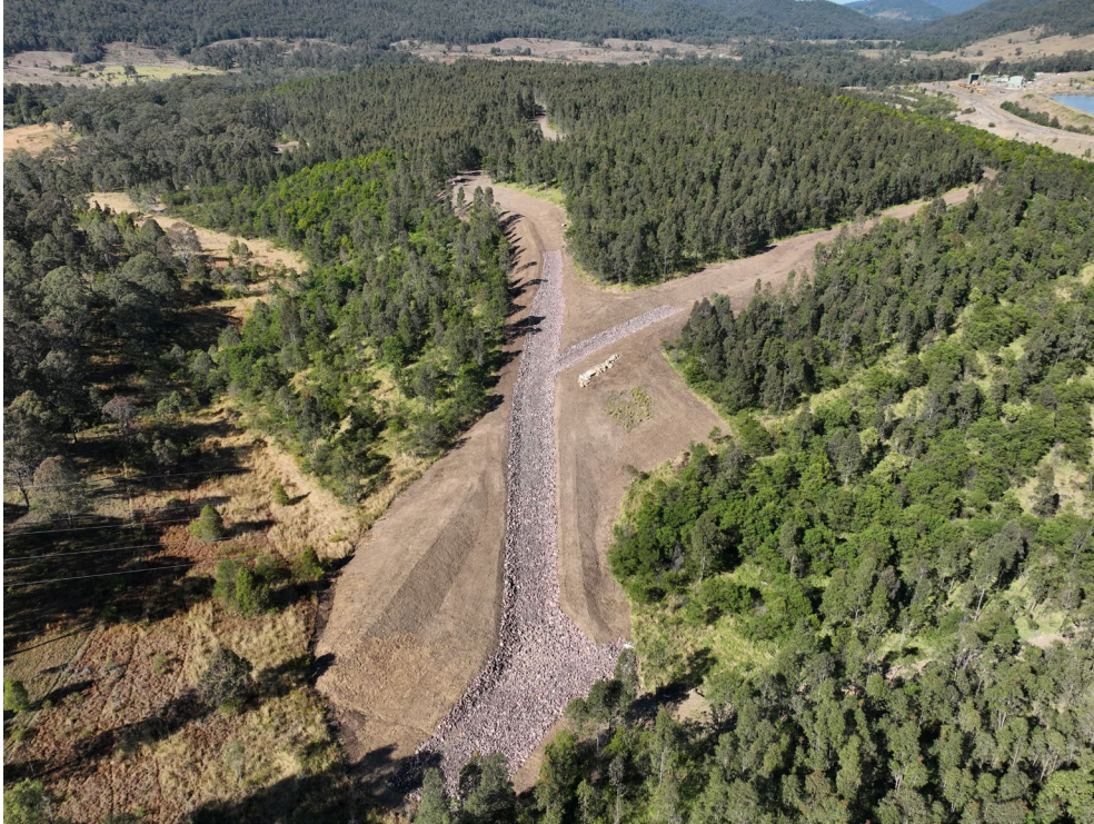
Photo: Completed rehabilitation crest drains, July 2025
