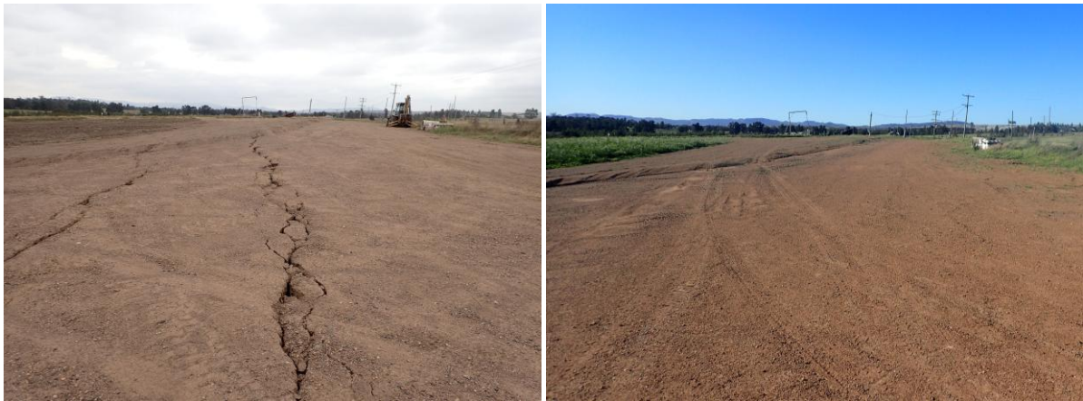
Photo 2: Example of subsidence cracking along stacked goaf edge and after crack remediation at the AUM
