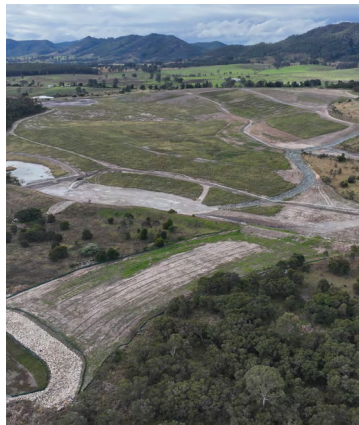
After Bowens Road North Open Cut Pit
