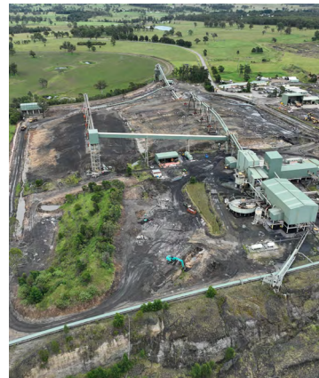
Before Coal Handling and Preparation Plant
