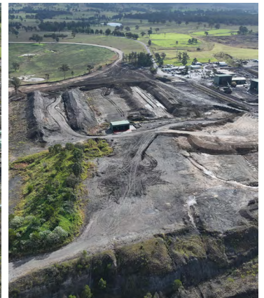
After Coal Handling and Preparation Plant
