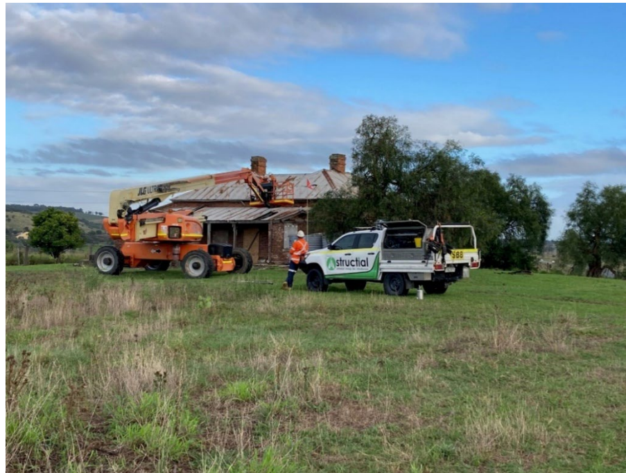
Roofing repairs being undertaken
