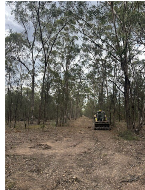
Mulched track near between airstrip and Cook House
