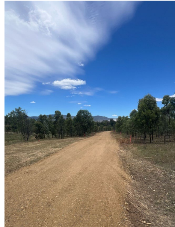
New section of access track
