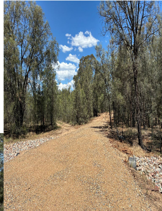
Rebuilt culvert and approaches
