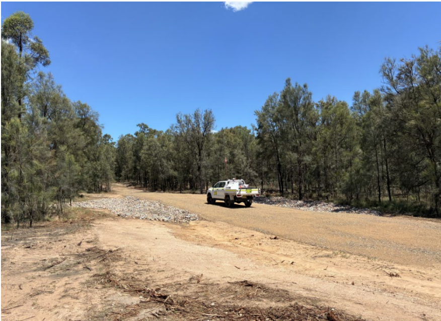
Rebuilt culvert and approaches
