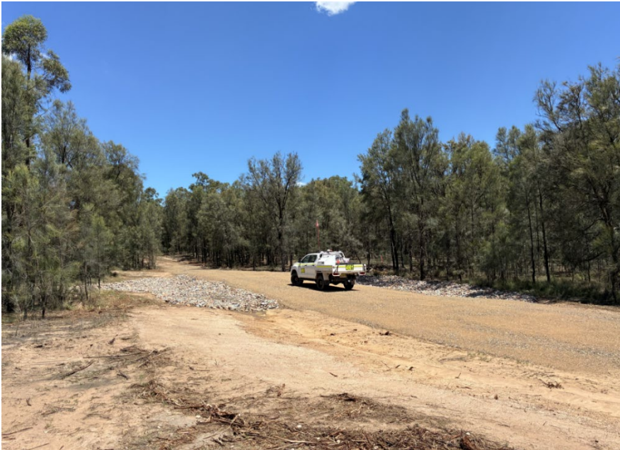
Rebuilt culvert and approaches
