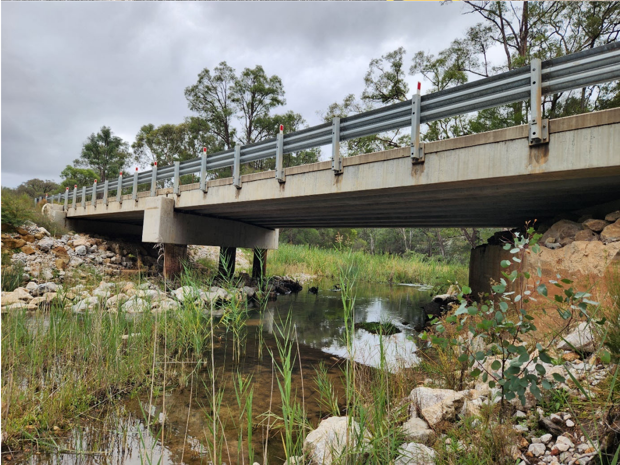
Fig. 6.1 Ulan Road bridge over Goulburn River
