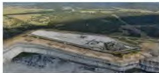
Longer section of West Pit South by April 2026
