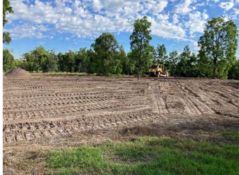
WSW topsoil spread across planting area, NBA
