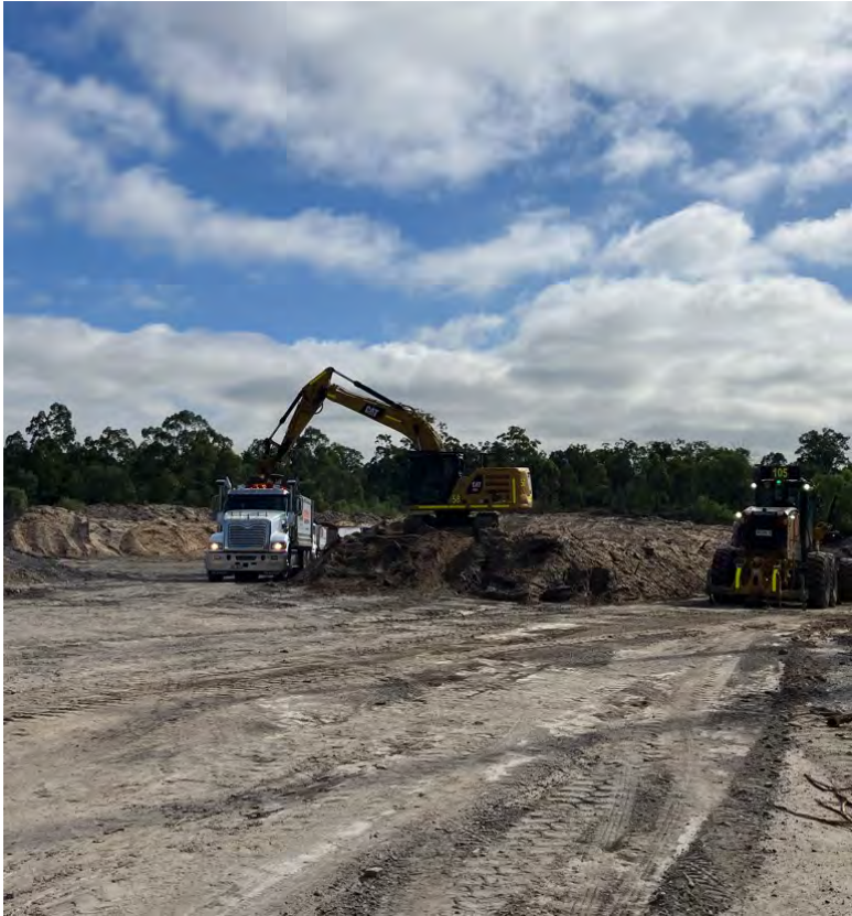
WSW topsoil loaded from WML stockpile for transport to NBA
