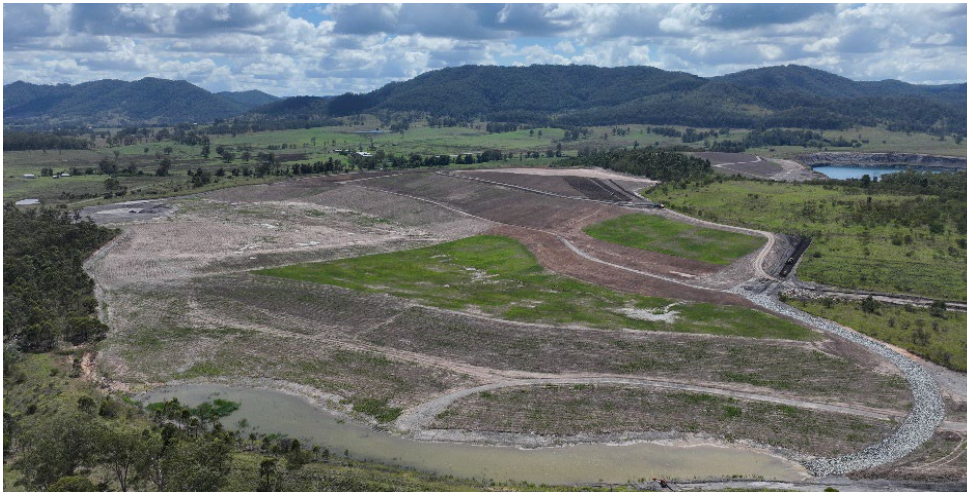
Plate 10: BRN Rehabilitation Progression, January 2025
