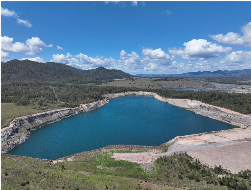
Plate 7: Avon North Void, looking south. January 2026.
