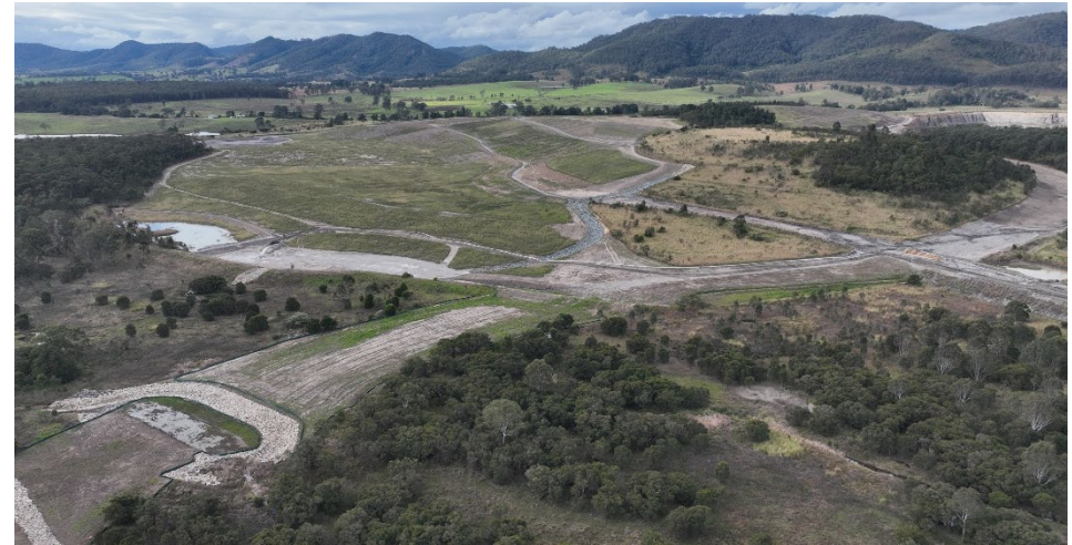
Plate 11: Completed BRN Rehabilitation, July 2026
