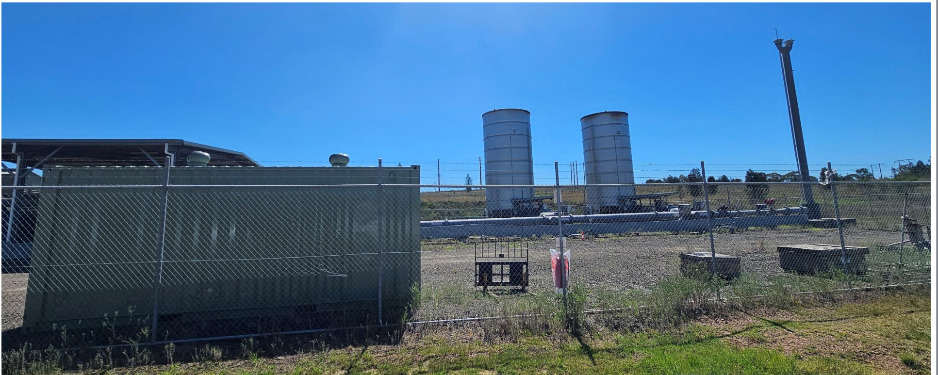
Plate 10 Central Gas Drainage Plant, including CGDP Flares
