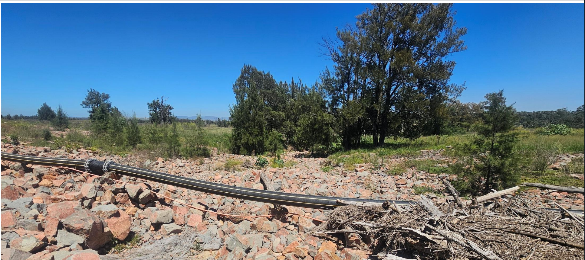
Plate 18 Bowmans Creek (Eastern) Diversion block bank, facing west
