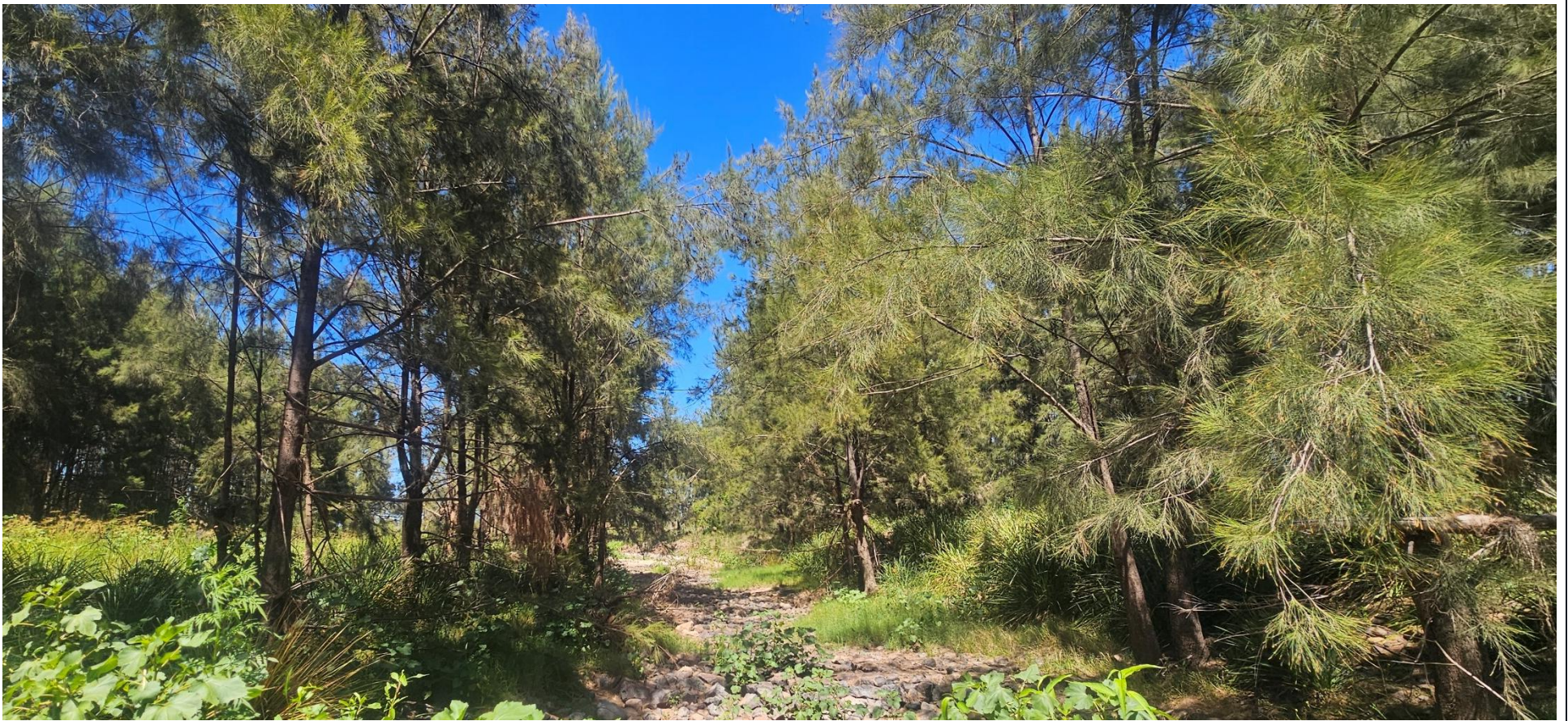
Plate 16 Bowmans Creek (Eastern) Diversion channel, facing south
