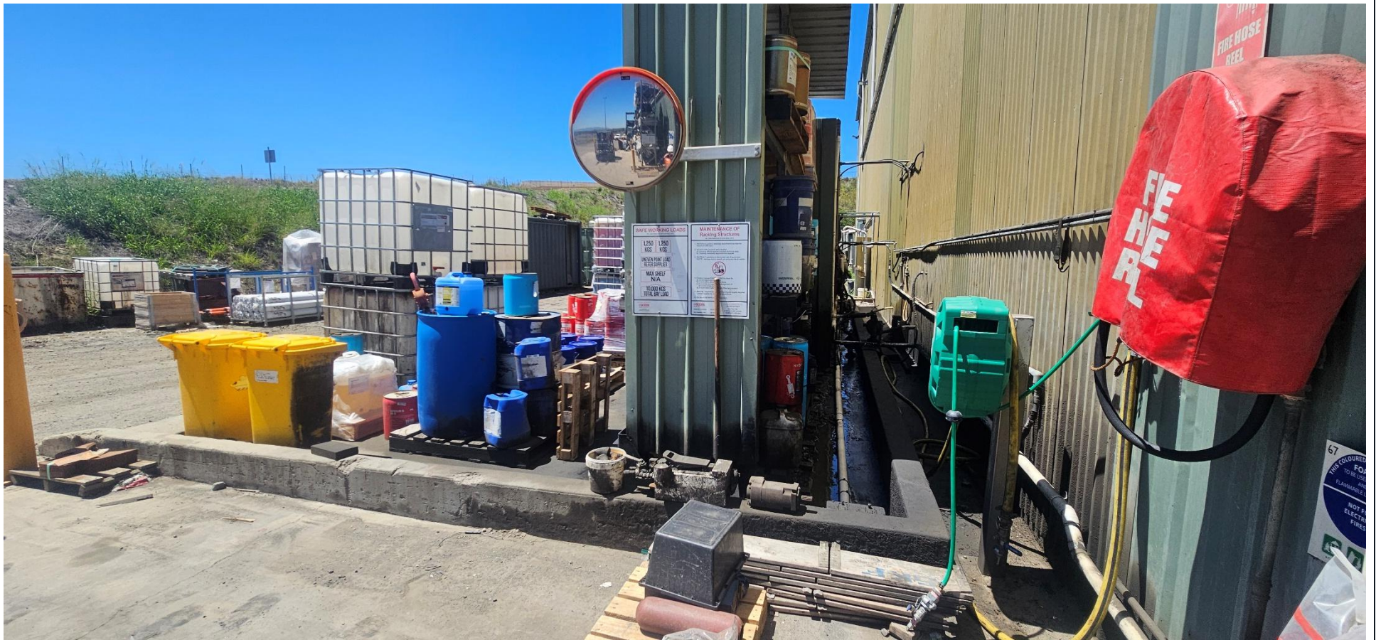
Plate 22 Bunded oil and chemical storage at the Mine workshop, including stocked spill kits
