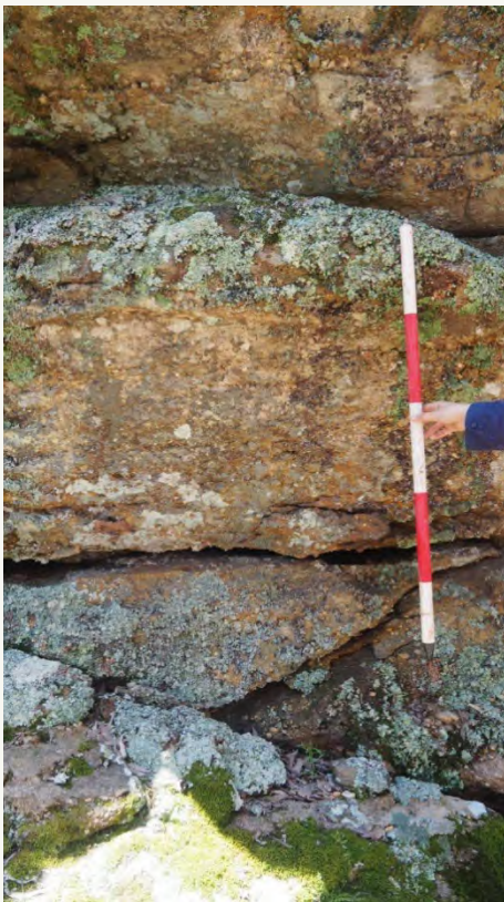
Plate 125: Close up of weathered sandstone at site S1MC491 (AHIMS ID# 36-3-3792), showing the salt/granular loss and microvegetals present. Photo taken on 2 December 2021.
